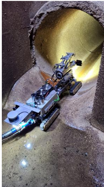
Figure 2: The SewerVUE's remotely-operated vehicle Multi-Sensor Inspection entering the pipe.
